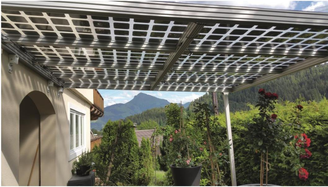
**Figure 12: Transparent Pv modules on Terrace**
