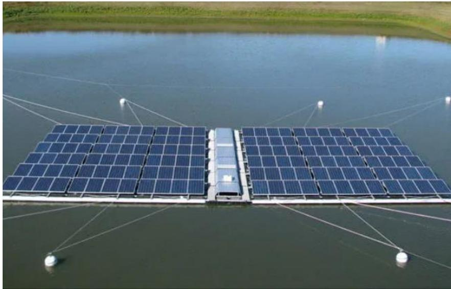
**Figure 23: Floating PV Systems for Aquafarming (CleanFuture, 2018)**
