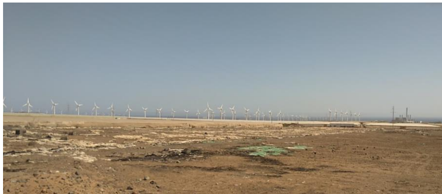
FIGURE 3.13 – VIEW OF THE PLANT OF LLANOS DE JUAN GRANDE
